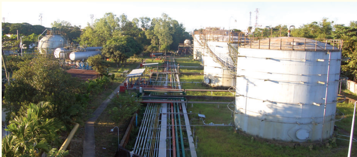
Kailashtila LPG Plant, Sylhet.
